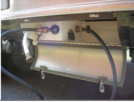
Hot and cold washer lines attached to hose bibs
