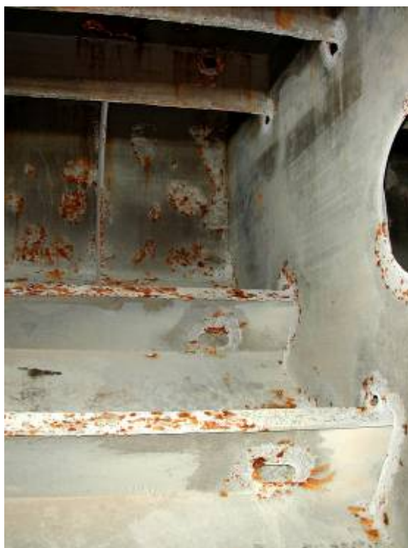
PHOTOGRAPH 4 Heavy Calcareous Deposits
