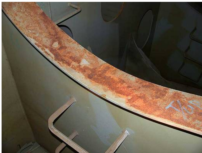
PHOTOGRAPH 7 Under Thickness
