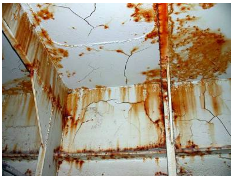
PHOTOGRAPH 25 Typical Mud Cracking in a Thick Coating
