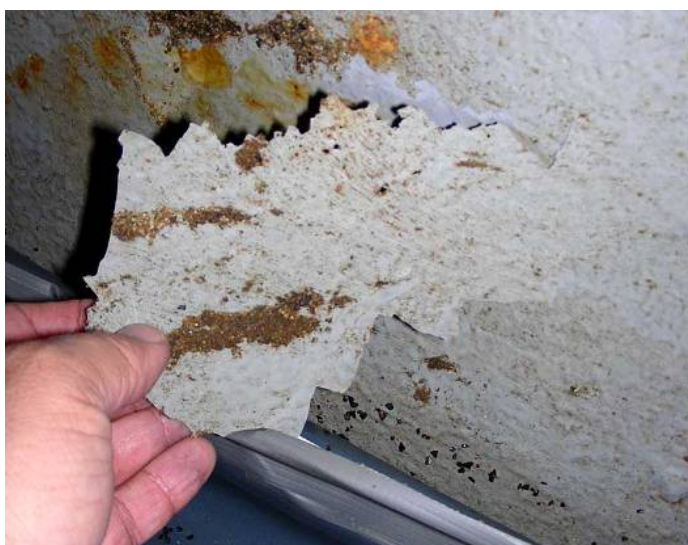
PHOTOGRAPH 6 Over Thickness
