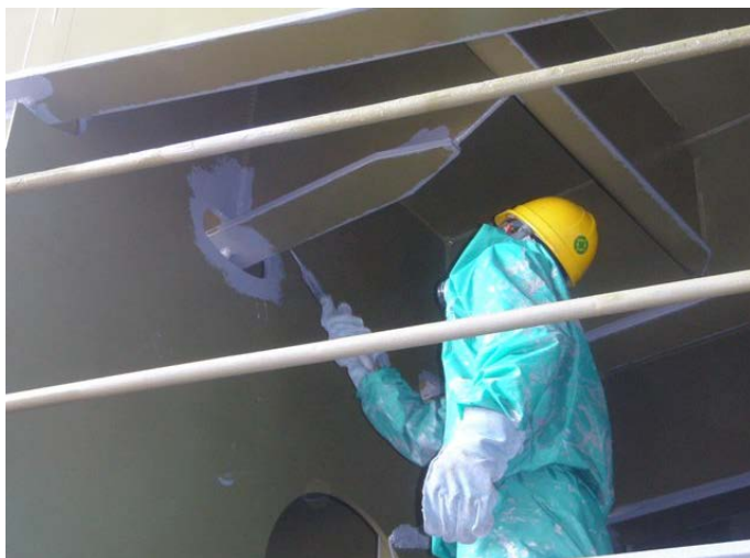
PHOTOGRAPH 18 Stripe Coating Application (1 January 2017)
