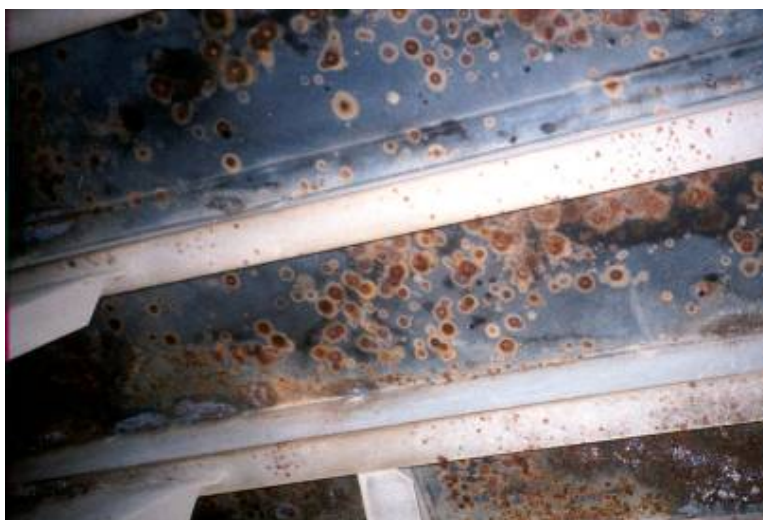
PHOTOGRAPH 10 Through Film Breakdown
