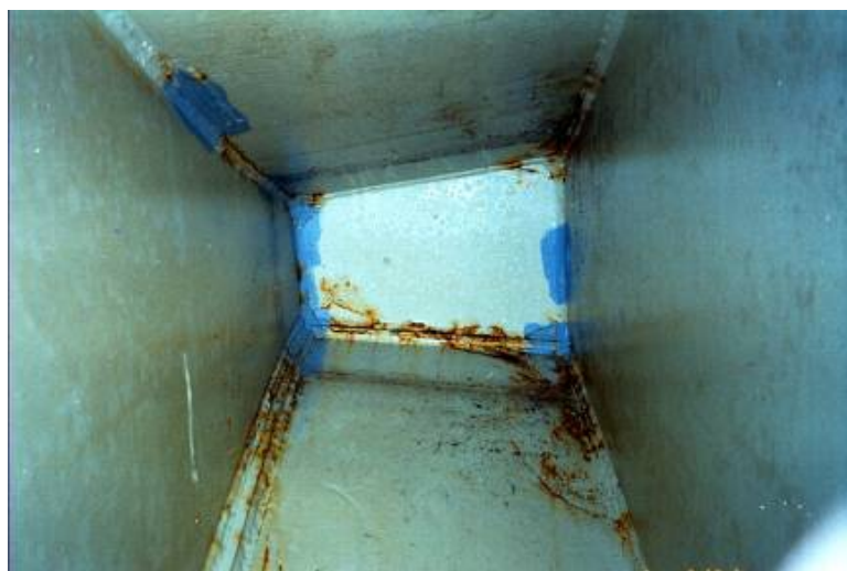
PHOTOGRAPH 19 Corrosion at Welds
