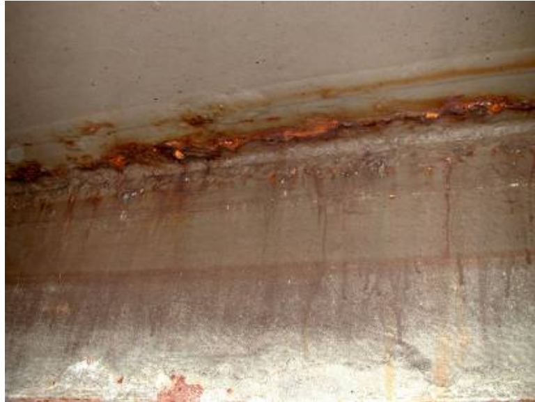
PHOTOGRAPH 18 Corrosion around Weld
