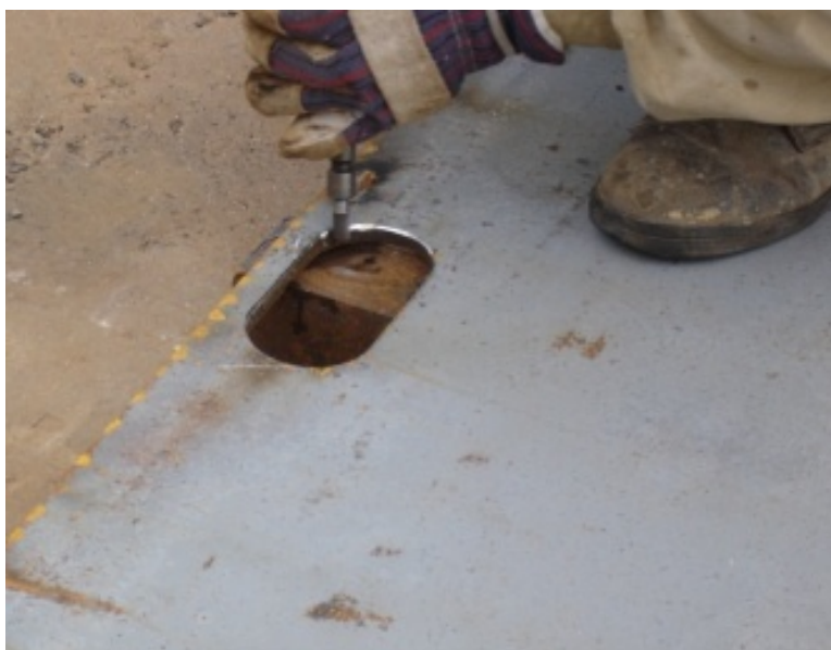
PHOTOGRAPH 14 Edge Preparation (1 January 2017)
