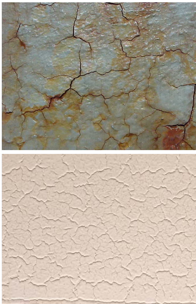
PHOTOGRAPH 4 Cracking (1 January 2017)
