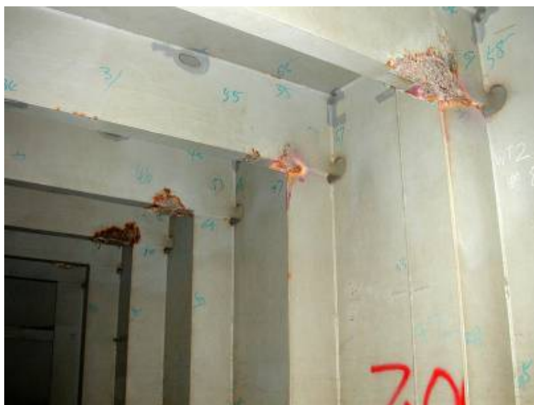
PHOTOGRAPH 26 Stress-induced Coating Failures
