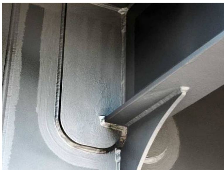
PHOTOGRAPH 2 Stripe Coating on Welded Details
