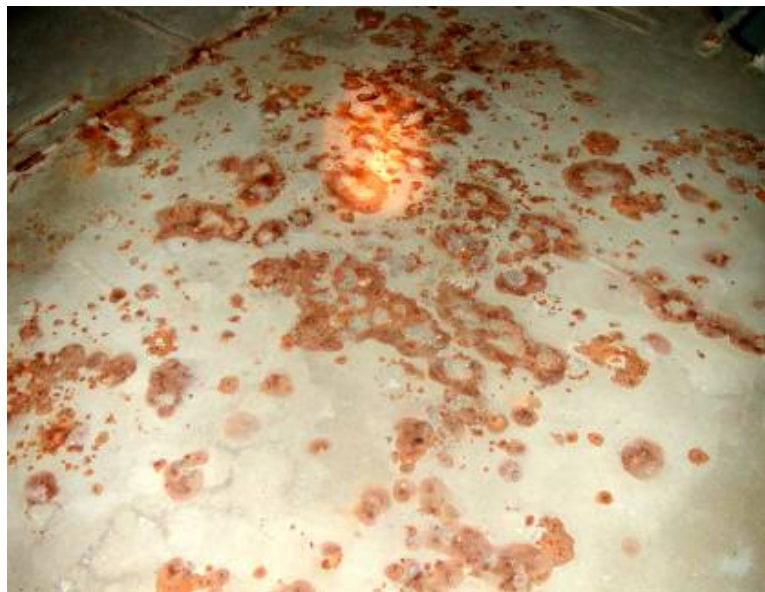
PHOTOGRAPH 12 Corrosion Spots on Stringer Deck
