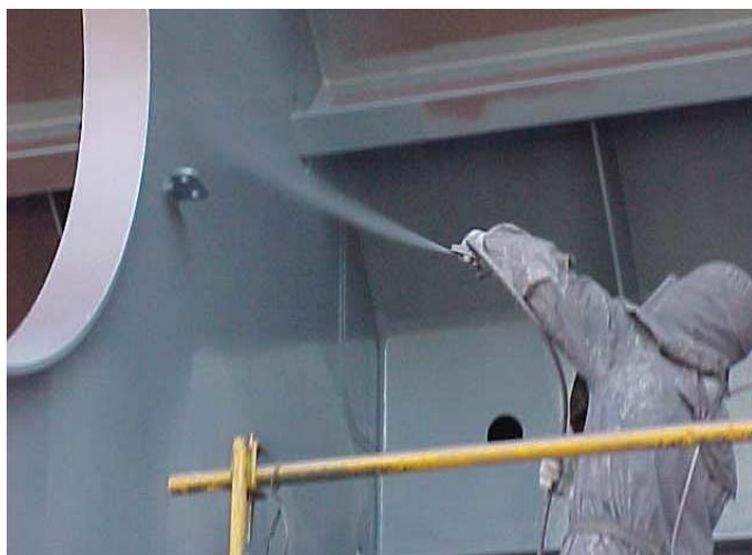
PHOTOGRAPH 19 Spray Coating Application (1 January 2017)
