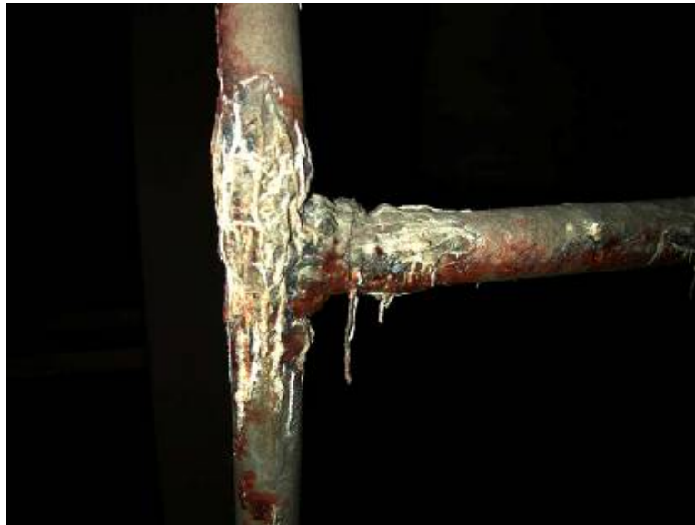
PHOTOGRAPH 21 Voluminous Calcareous Deposits
