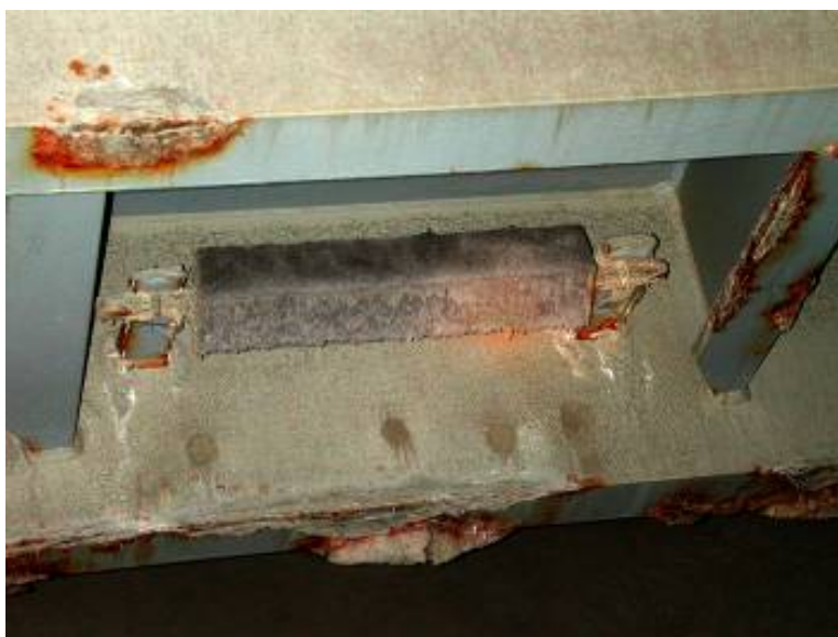
PHOTOGRAPH 5 Poorly Sited Anode
