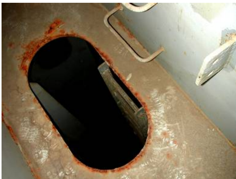
PHOTOGRAPH 17 Coating Breakdown around Cut Out
