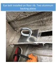
The eye bolt uses two backing plates that capture the rib. Once the batteries were installed, it was gravely evident that the coach sheet metal would flex a very noticeable amount. It is no wonder that these rivets may pull out under the dynamic load of these heavier batteries. Add compromised holes, lower strength rivets or poor riveting techniques and "battery detaches on the highway".
