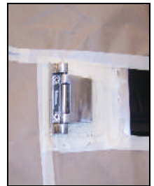
Figure 2: mask the door hinge
