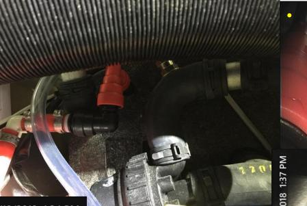
T-fitting off of hot wat leaking
