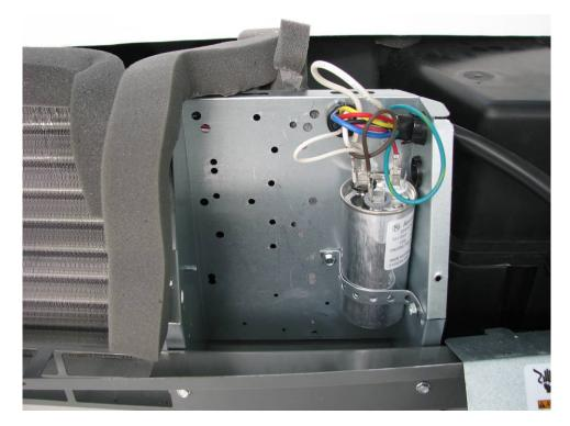
I removed the PTCR start assist by pulling it out of its bracket and then unscrewing the mounting screw. As you can see in the picture, there was lots of room to mount the SmartStart in the box.
