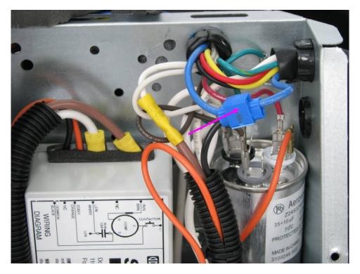
I then cut the spade connector off the black wire and used a 14 gauge tap splice connector to make the connection to the blue wire. Another, and perhaps better, way to do this would have been to cut the blue wire and attach the black wire to the resulting 2 blue wires ends using a closed end crimp connector.
