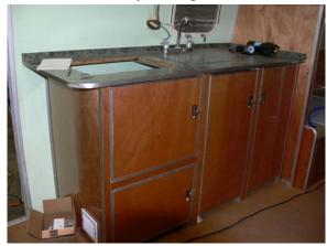
Kitchen sink cabinet has a newly added door where the oven used to reside. Smaller door below gains access to the New Suburban 35000 BTU Furnace. Sink countertop is made out of 3/4" plywood which was sealed and varnished at all sides. Formica counter top has a laid back backsplash. Face edges are trimmed with anodized aluminum T trim. Open cut out is where SS cook top will be installed.
