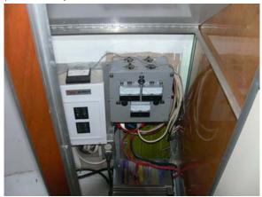
Both, Positive and Negative battery leads are protected by 50 Amp Circuit Breakers. On top of the 110 Volt panel box is a Blue Sea AC Analog Voltmeter. Two Blue Sea DC Analog Voltmeters and one Analog Amp Meter below them, occupies the face of 12 Volt panel. PERKO, dual battery switch is mounted right below, [and only partially visible in the picture].
