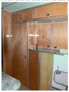
All cabinetry is made from 4mm OKUME Marine Plywood. Counter top above the Fridge is also made from the same as the kitchen counter top. To the right of the bedroom wall is the hanging closet. Note the cabinet with shelves above unoccupied fridge space, and the utensil cabinet with three new drawers behind the door and storage underneath, between the closet and fridge space.
