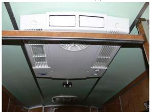
A new Low Profile 15000 BTU Carrier AC with a heat unit was installed in January 2008. Rectangular frame was cut at 45 degrees and was first inserted in pieces and riveted into AC opening in the roof. Corners of the mounting frame were TIG welded then for added rigidity to the roof area. Condensation drain tube was already in the wall, but I had to special order a \$0.90 drain elbow, which should have been supplied with a unit. For the interior doors we have ordered a accordion doors.
