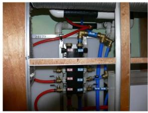
Water system is made entirely from PEX tubing and brass fittings. Manifold is mounted onto a welded Gray Tank retaining frame, which is located under the kitchen sink. Shut off valves are provided for each water line. Blue tank is presently being professionally cleaned and will be connected to already existing PEX line.
