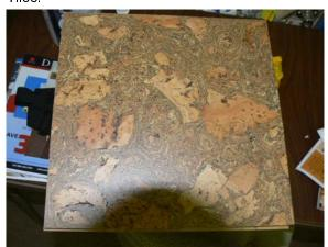
Cork tile has brown and Earth green hues which will match the Sea Foam green walls as well as the kitchen countertops. Only exposed to view area will be tiled. Cork under-layment was sealed and varnished after installation.
