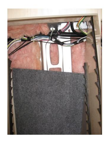
Using your hand, feel the area behind the shower. There is an aluminum panel about 3" from the top. The wires must go in front of the panel. Push the wires down to the area below where the access panel is located.
