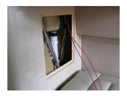
Reach up and grab the wires and pull them down, then open the folding seat, and route them near the wall under the seat toward the area below the cupholder. Use zip ties to secure the wires both behind the shower, in the compartment above the seat as well as below seat.
